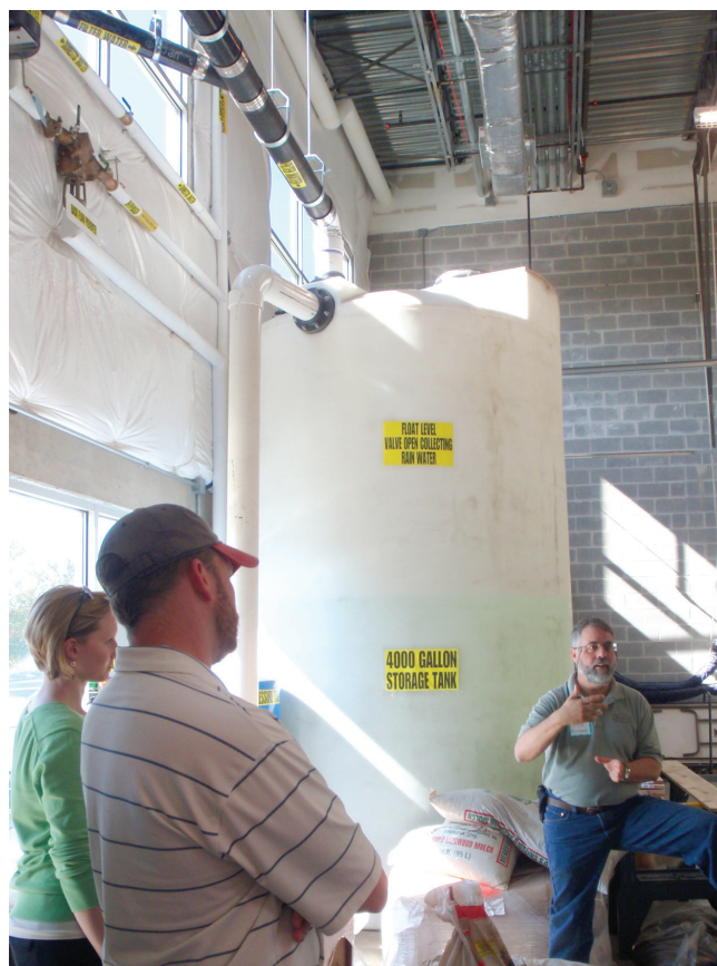
Figure 1. Typical RWH system.
